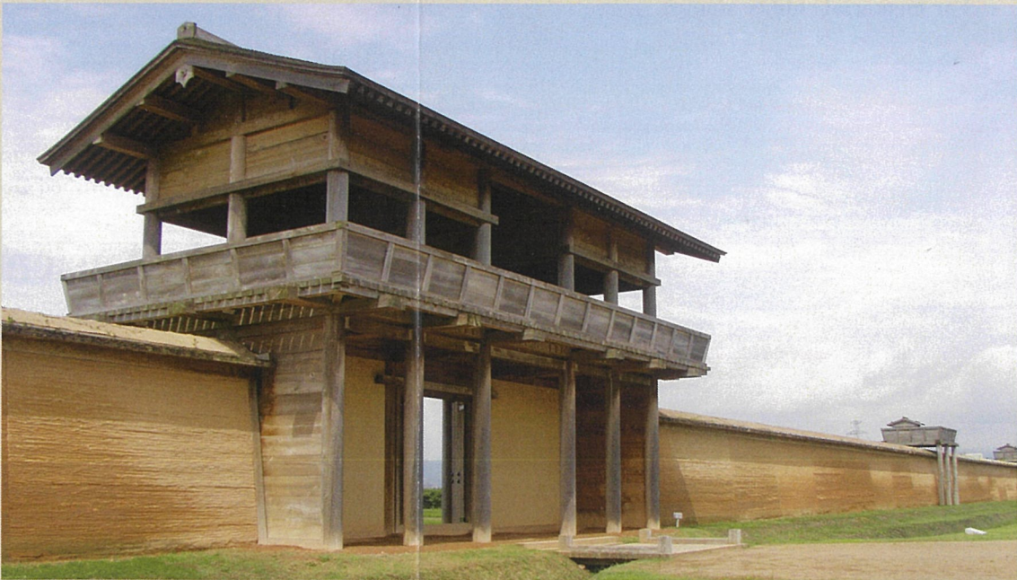
South Gate of the outer wall, earthen wall, and watchtowers
